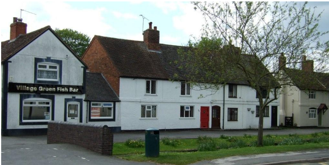
Photograph 3 Village greens providing the foreground to buildings
