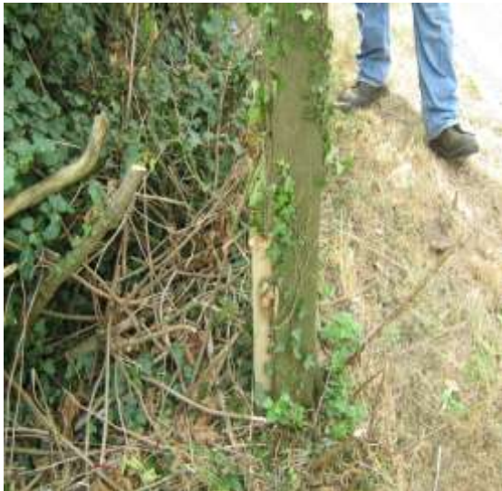
Footpath R133 – loose way marker post - repaired.
