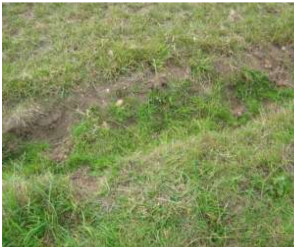
Footpath R135 – the rut that could be trip hazard
