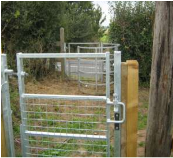
Footpath R135 - the new pedestrian gate looking back towards the Fosse Way and existing kissing gate
