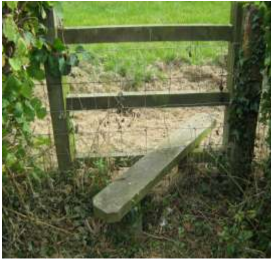
Footpath R133 - far side of Fosse - top step nailed.
