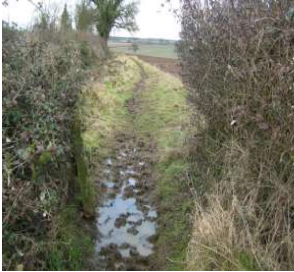
R132x Bridleway – Wooden gate now missing.
